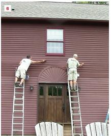
Festool CT Midi HEPA Dust Extractors, we worked our way up toward the soffit (1), sanding off most of the finish (2). The pitting was random in intensity and location, and a small return wall adjacent to the front facade needed only to be scuff-sanded (3).
