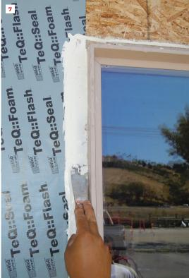
Here's why I prefer method "B." Sealant under the nailing flange is a critical detail for keeping water out. But with the "A" methods, this detail is covered up when the flange is flashed, and so is difficult to inspect (1). The "B" methods allow for a more complete inspection by superintendents, who look for "squeeze-out" to verify that the sealant has been correctly applied (2).
