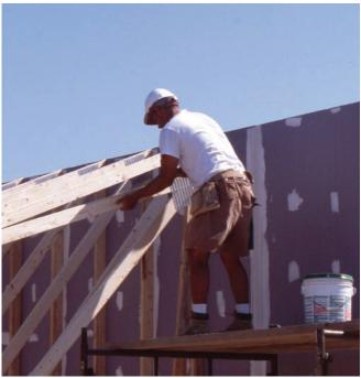
The author's crew frames a duplex building with units arranged back-to-back (see illustration, facing page). Working from a rolling scaffold on the floor slab, the crew first attaches  $\frac{5}{8}$ -inch Type X gypsum board to the unit separation stud wall (above left), then sets trusses for the roof (above right).
