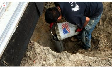
Left: When the helical piles have been driven to the required depth, the crew pushes a PVC grouting tube into the ground around the shaft. The top of the pipe is then cut off 4 to 6 inches below the top of the pile shaft (4). After the sand is cleaned out of the tube with a high-pressure water jet, the pipe is filled with cementitious grout (5).
