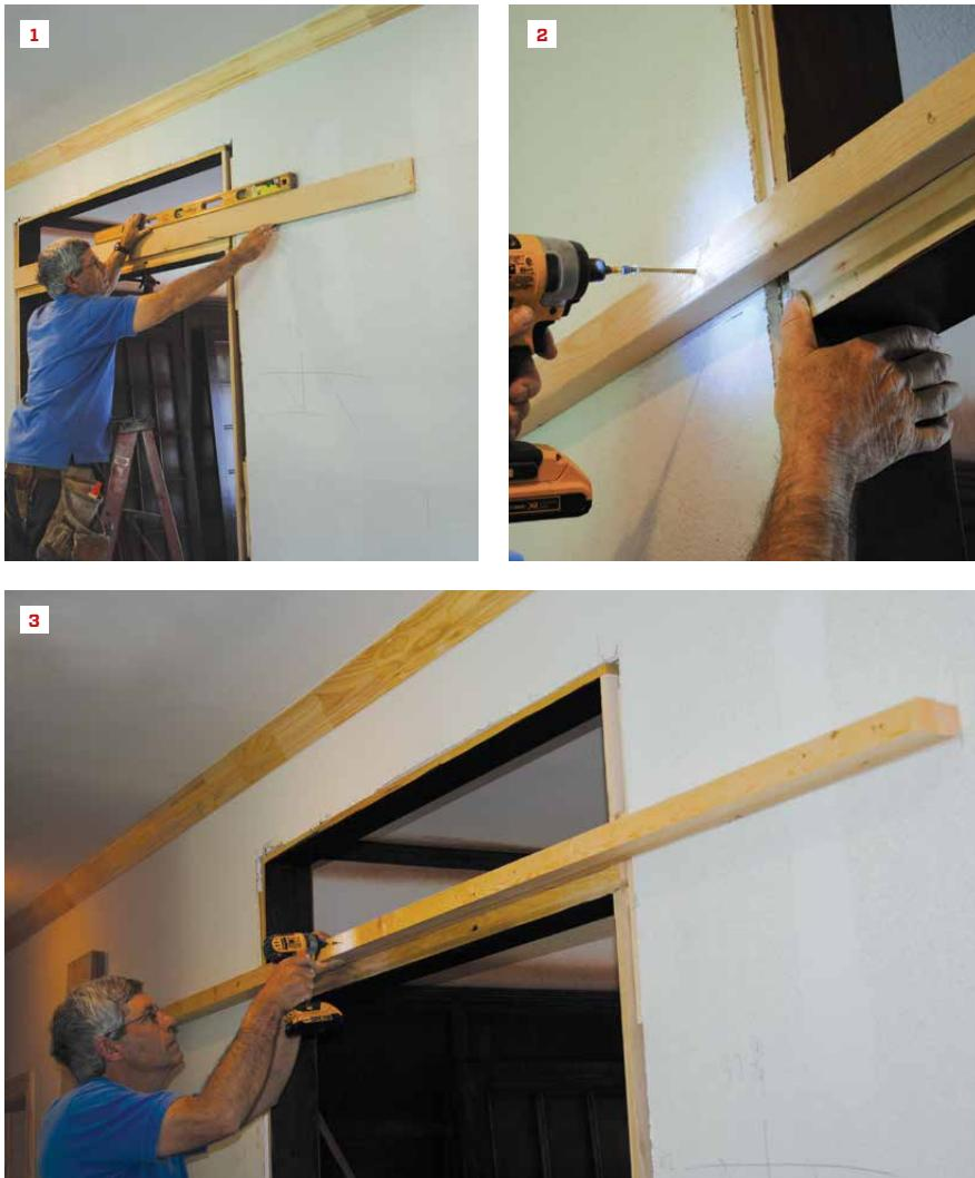
In preparation for mounting the track for the barn-style doors, the author drew a level line across the opening and onto the walls at the appropriate height (1). He then ripped a 2x6 in half and, using his line as a reference, centered the first piece on the opening and screwed it to the wall framing (2). Screwing the second ripped piece to the first with the bottom edges flush to each other (3) created a 3-inch-wide header to attach the track to.
