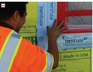
**Seal side-flashing edge.** For added protection, apply a bead of sealant along the edge of the side flashing where it butts into the window frame. This will help if the SAF does not adhere properly to the nail fin because of dust, cold, or moisture **(23)**. Tool the sealant bead with a finger. The sealant helps mitigate potential moisture entry points from wrinkles in the side flashing **(24)**.
