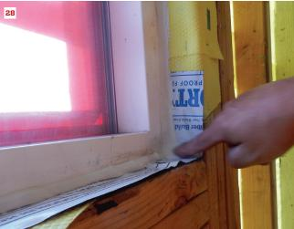
**Seal the interior.** On the inside of the window, apply a bead of sealant 6 to 8 inches down each side and all the way across the bottom (27). Tool the sealant into place using a finger. This will stop any unintended water from reaching inside the home. Apply low-expansion foam around the rest of the RO (28).
