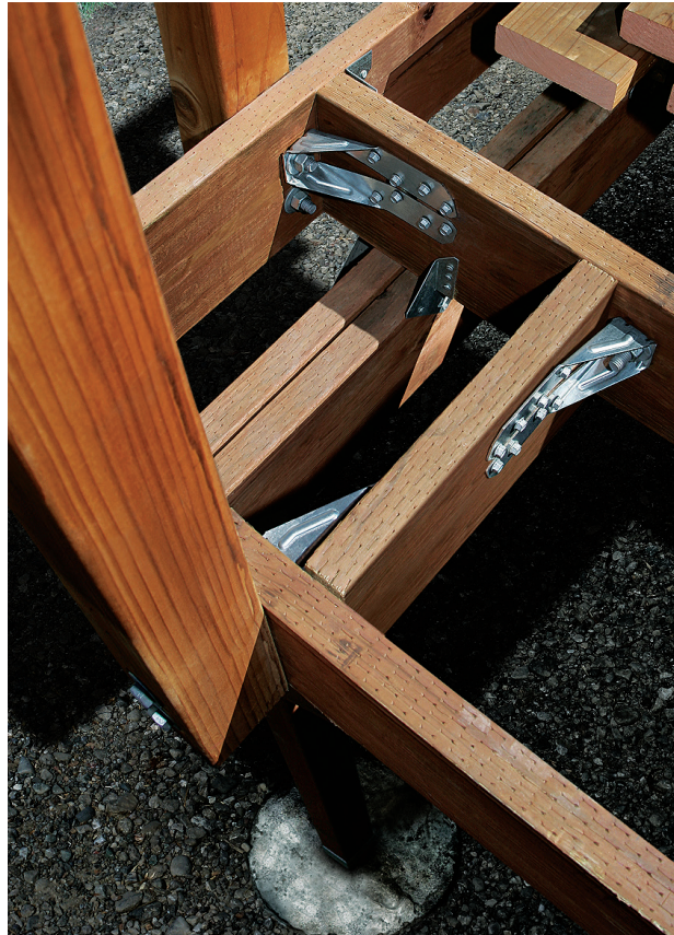
Shown here is a code-compliant guard-post-connection detail made using Simpson Strong-Tie DTT2Z deck post connectors ( strongtie.com ).
