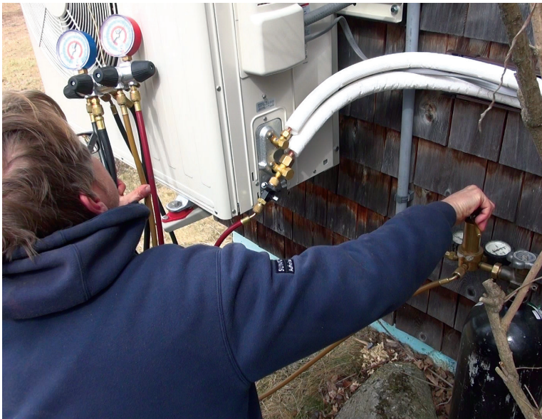
ReVision Energy tech Dave Ragsdale sets up equipment for the pressure test and triple-evacuation refrigerant-line-clearing procedure for a newly installed Mitsubishi mini-split at a rural home in Maine.
