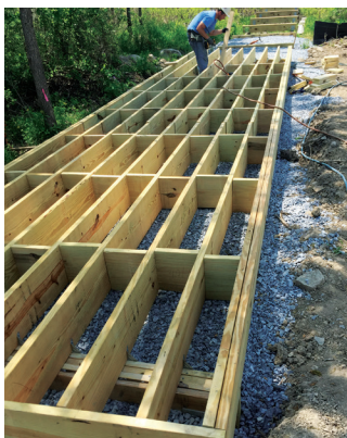
Figure 6. The framing consisted of 2x12s at 12 inches on-center, with bridging between joists every 4 feet on-center. The joists were supported by 6x12 beams located on 12-foot intervals.
