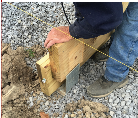
Figure 5. Because the four-ply beams were too wide to fit into the 6 1/8-inch-wide U-shaped brackets on top of the helical piles, 1/8-inch-deep mortises needed to be routed at the ends of each beam.
