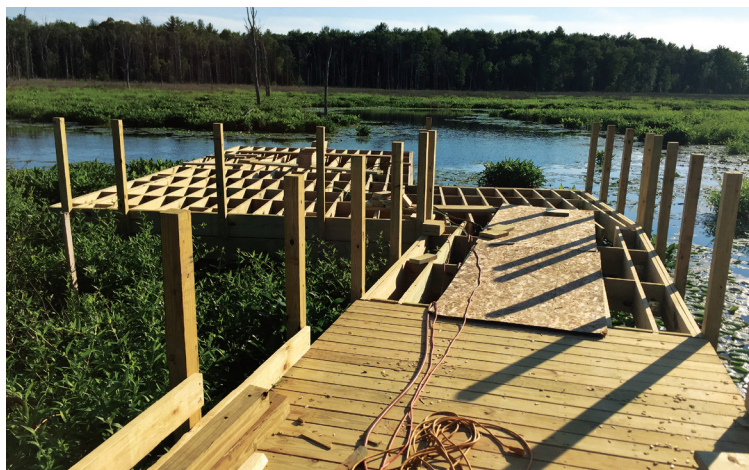
Figure 9. The boardwalk terminates in a 24-foot-by-30-foot observation platform, as well as a floating boat launch.
