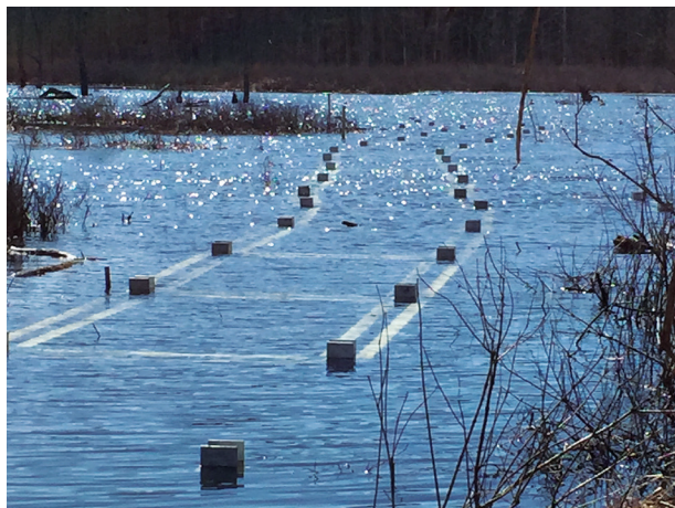
Figure 4. When the snow melted in the spring, the water level in Round Lake and Anthony Kill temporarily rose to the level of the anchor brackets.
