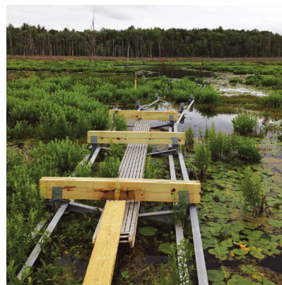
Figure 7. The crew installed decking as they framed the boardwalk, enhancing access with aluminum planks.
