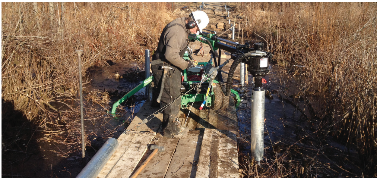
Figure 1. A worker from Techno Metal Post of Albany installs one of the helical piles that were used to support the boardwalk framing in the sensitive wetlands.
