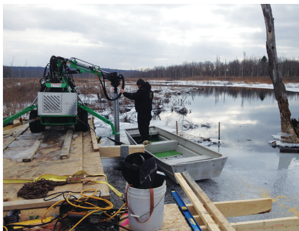
Figure 2. Conditions became more difficult as the project moved into deeper water (left). Once winter arrived and the wetlands froze over, it was actually easier to position and install the piles (right).
