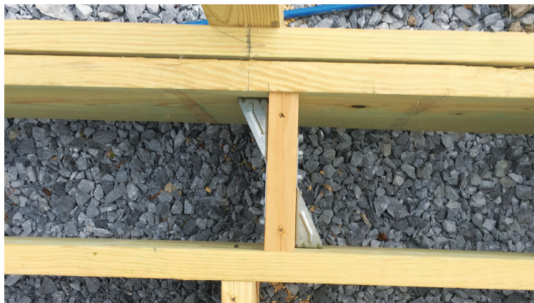
Figure 8. Simpson Strong-Tie DTT2Z brackets were used to secure the 42-inch-high handrail posts to the framing. The posts are located 4 feet on-center.
