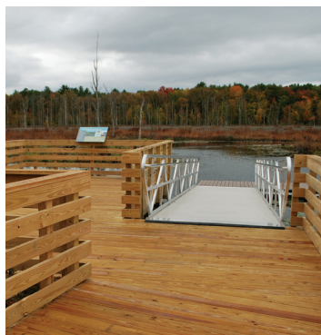
Figure 10. The rail system consists of 2x6s face-nailed to the posts, and a continuous 2x6 top rail. A 7-foot-wide aluminum gangplank leads to the floating boat launch.
