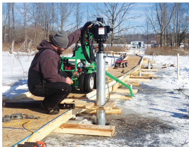
Figure 2. Conditions became more difficult as the project moved into deeper water (left). Once winter arrived and the wetlands froze over, it was actually easier to position and install the piles (right).
