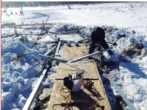
Figure 3. Once the 2-inch-diameter piles were in place, the crew cut them to length and installed the galvanized anchor brackets. The structure was reinforced with L4x4x1/2 steel cross-bracing welded to the piles.
