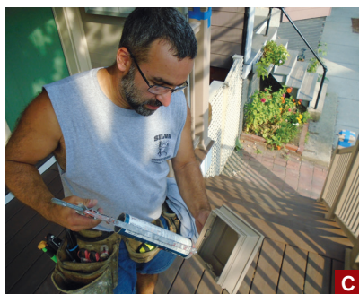
The upper beams are screwed to the posts (A), then the upper rails are snapped into place (B). To prevent the post caps from being dislodged, the author glues them to the post sleeves with elastomeric sealant (C). Masking tape holds the post caps in place while the sealant cures (D).
