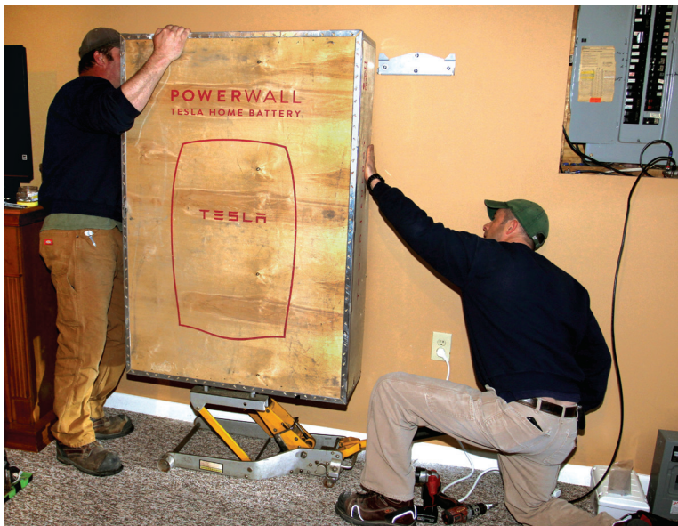
Electricians Brian Ritz (left) and Scott Millette (right) use a floor jack to maneuver a 214-pound Powerwall unit into place in a Vermont home. The battery is only rated for temperatures down to -10°F, so it can't face Vermont winters outdoors.
