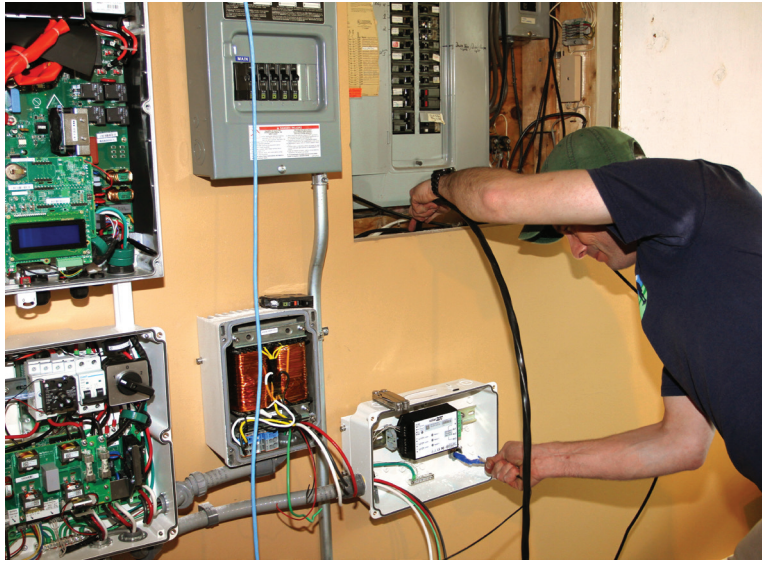
Scott Millette pulls cable into the smart meter box from the home's main panel. To the left of the panel is the load center with breakers serving the home's backed-up circuits.
