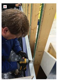
Paisley uses metal screws to pin the H-studs and C-channel to the gypsum board (4, 5). At each stud location, he places a heat-softenable breakaway aluminum clip (6). He then screws the clip to the C-channel (7) and to the stud (8). If a fire should cause a structural collapse on one side of the wall, the clips would melt and allow the wood to fall away, leaving the firewall intact to protect the other building.
