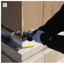
To rough-cut a shingle to the scribe line, first score it with a razor knife (6), then snap off the waste (7). When the shingle is fastened in place, fine-tune the edge with a block plane, holding it flat against the adjacent shingle (8). A 6d stainless steel finish nail, driven through the edge and set, finishes the joint (9).
