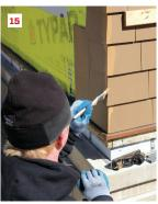
A level line guides each following course (10). Trim shingles in place using a razor knife (11) and a block plane. A corner notch lets the top courses slip into a rabbet in the trim above (12). At the top, the cutting is completed with a knife (13). The top course is hand-nailed (14). A coat of matching stain finishes the corner (15).
