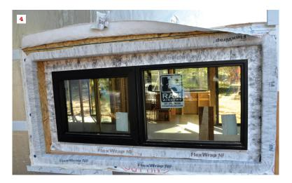
To remedy the botched window job on his site, the author worked with the local Tyvek distributor. The housewrap was peeled back and FlexWrap applied along the edges of the recessed opening and over the window flanges (4). Next, Tyvek Flashing and Joint Compound is gun-applied into the corners (5), followed by a second, more fluid product—Tyvek Brush Formulation (6)—to create a seamless membrane around the entire window.
