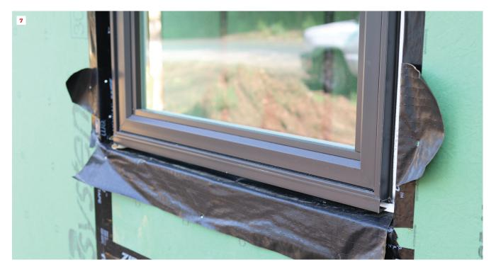
**Unsure of what to do on a Zip System wall,** a builder simply installed wide pieces of a paper-and-plastic-laminated flashing tape, which he planned to secure with Zip System sheathing tape. This detail would likely have deteriorated quickly and become a homeowner's nightmare. With almost no roof overhang on this house, these openings will be exposed to a deluge of water.
