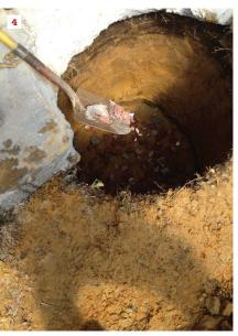
The new footings will straddle the existing slab, so part of it needs to be removed to allow access to excavate the holes. First, the author traces the footing's perimeter onto the slab (1) and removes the concrete using a jackhammer and sledge (2). Then he digs the footing hole to its required depth (3). Because of the high water table, the hole had to be pumped as it was dug. In the bottom of the hole, a layer of crushed stone will support the footing and keep the pump clear of the soil (4).
