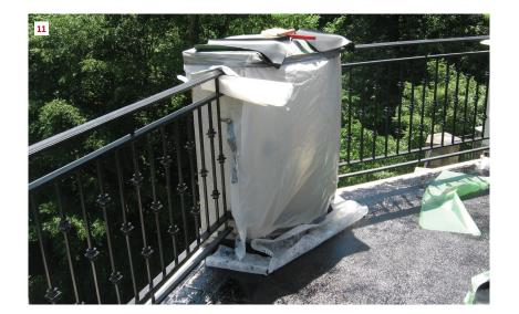
The rubberized asphalt membrane is applied hot, and splashes or drips will stick to anything and are a hassle to clean up. At left, the crew has protected the masonry rail posts with poly (11). Over the reinforced membrane, the crew lays a dimpled plastic drainage sheet with filter faces, then builds up a mortar bed reinforced with galvanized wire mesh (12). Finally, they set new stone pavers into the wet mortar (13).
