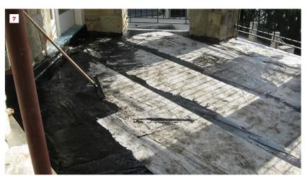
then a piece of coil stock flashing was placed on top and bent up the wall. Housewrap on the wall was tucked behind this flashing instead of in front as it should have been, but that probably didn't matter—because water was free to run across the waterproofing and into the wall underneath the aluminum flashing. Also, aluminum flashing will corrode in contact with masonry. That process was well underway in exposed areas.
