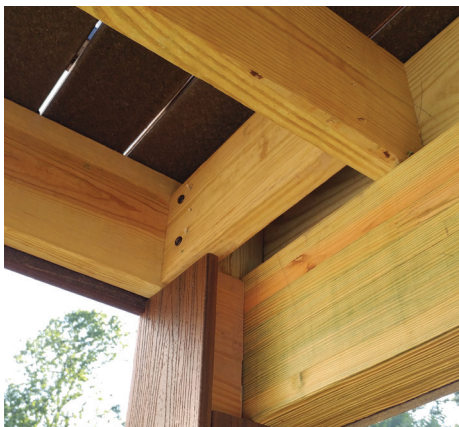
Figure 3. Blocking between joists at the outside corner allows the post to be securely locked in place. Structural lag screws are used to make the connections between the posts, joists, and blocking.
