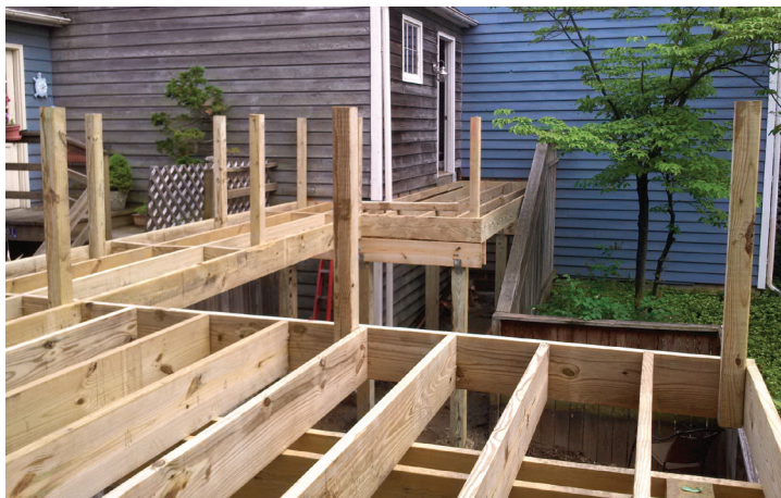
Figure 1. For most decks, the author installs the posts within the perimeter of the framing. Here, the posts have been tacked in place and are awaiting the installation of blocking.
