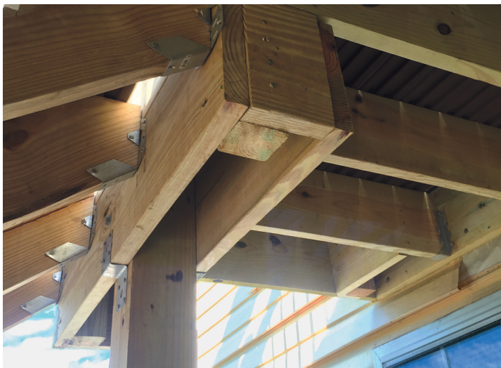
Figure 10. Additional blocking has been added to the dropped stair stringer header to reinforce the upper stair-guard-post connections.
