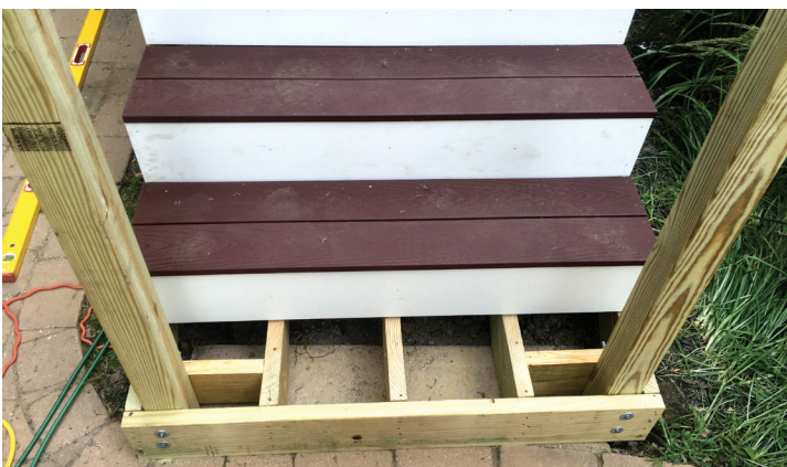
Figure 11. Stair stringers rest on a concrete pad and are fastened to the 2-by subriser and blocking with structural screws. The posts are then through-bolted to the assembly.
