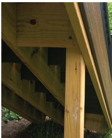
Figure 8. Blocking between stringers helps strengthen the stairs at guard-post locations, especially on longer stair runs.
