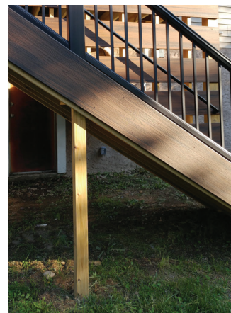
Figure 9. Additional support is provided by extending intermediate guard posts down to frost-protected concrete footings.
