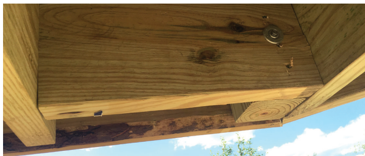
Figure 7. Posts that are located at corners can create leverage that tends to pull the framing apart unless there is additional blocking to reinforce the connection.
