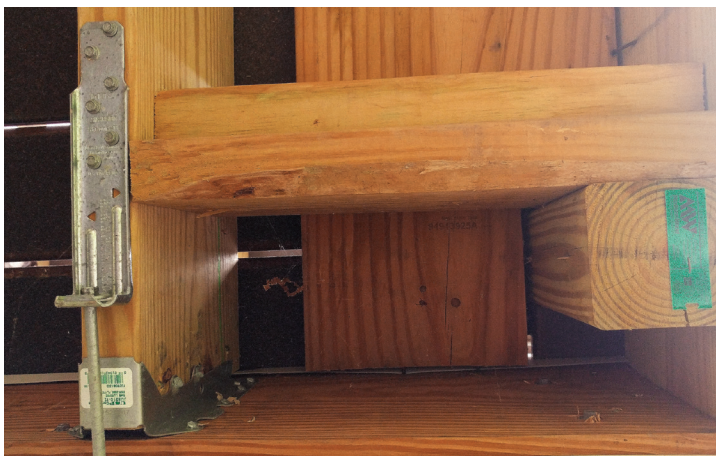
Figure 6. Inside corner posts are typically spaced away from the ledger, so the author installs blocking between joists as shown to reinforce the connection. Though not yet installed, blocking will later be added to fill the gap between the ledger and the post.
