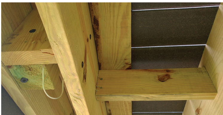
Figure 5. Carrying the blocking back an additional joist bay helps reinforce the rail-post assembly and prevent the side rim joist from rotating.
