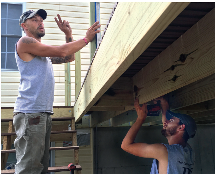
Figure 4. Blocking strengthens the framing where the joists run parallel to each other, such as along the side of the deck.
