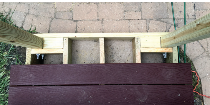
Figure 12. Blocking installed on the flat helps lock the corner posts in place and provides backing for decking that is cut to fit around the posts.
