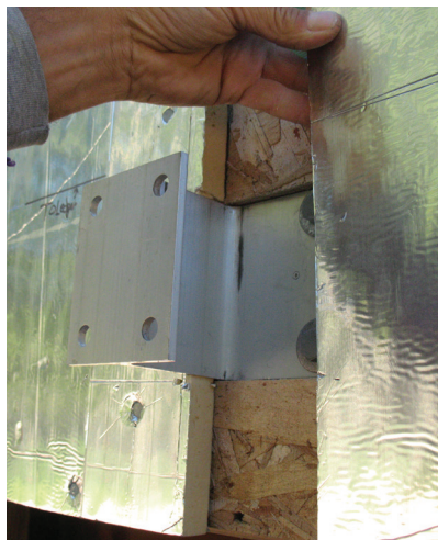
Figure 2. The foam panel is cut to fit around the bracket web. The brackets can accommodate foam up to 3 inches thick.
