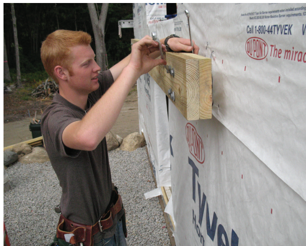
Figure 5. The ledger is a double 2-by that's through-bolted to the outside flanges of the brackets. Bracket spacing is determined according to the manufacturer's specifications and the loads on the deck.
