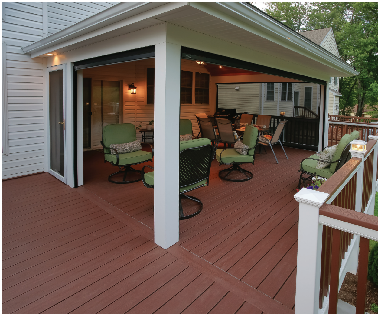
Figure 1. While fixed screen panels would create boundaries between the people using the porch and the adjacent deck, motorized retractable screens can quickly be used to remove those barriers when insects and weather conditions allow. A separate screen door is still required for regular access to the deck from the porch.
