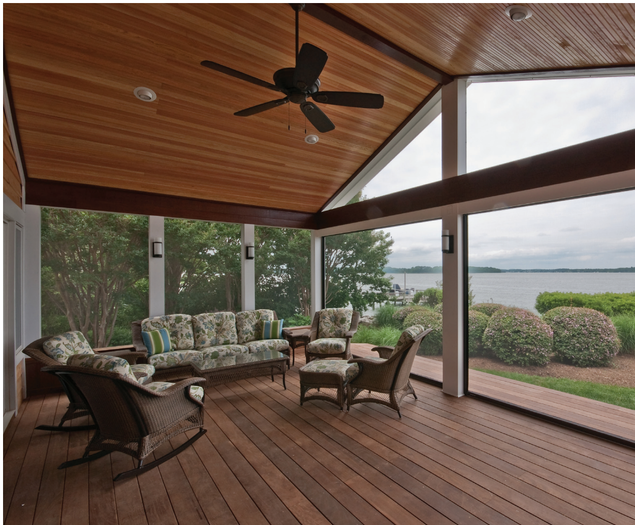
Figure 2. One major advantage of a retractable screen is that it can be used on an opening as wide as 24 feet, eliminating the intermediate posts that are needed for fixed screens and that would otherwise interrupt the view. It is also less expensive to frame and trim one large opening than several smaller openings.
