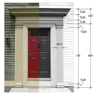
The heights of each architectural element within a specific classical order derive from D, the diameter of the column (width of the pilaster). For this Doric entry, column height should be 8D; the entablature 2D. Within the entablature (from top to bottom), the cornice is  $^{3}$ /4D; the frieze  $^{3}$ /4D; the architrave  $^{1}$ /2D.
