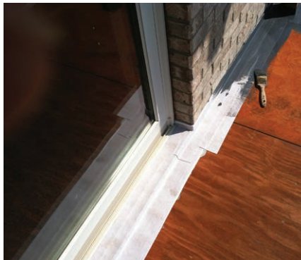
Figure 6. After flashing the joint between the deck and the wall with aluminum, the author sealed the metal flashing to the plywood with self-adhesive seam tape.
