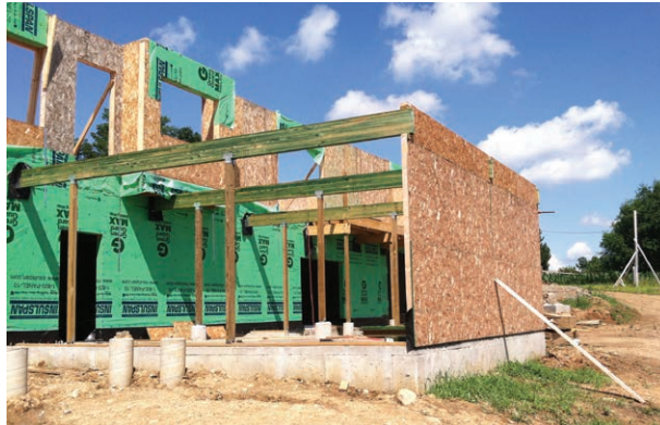
Figure 1. Three treated glulam beams provide the main structural support for the deck.
