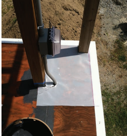
Figure 5. Patches cut from the polyester fabric supplied with the system were used to flash the guard posts and other penetrations through the roof deck.
