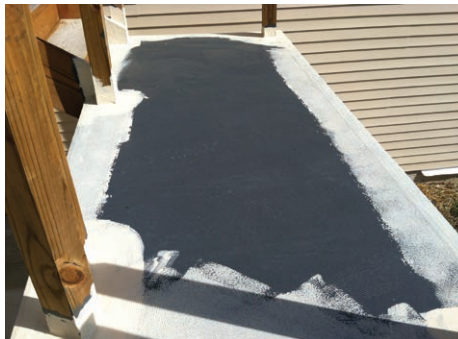
Figure 10. After the final coat of waterproofing cured, the author began applying the first of two coats of Safe-T-Deck top coating.
