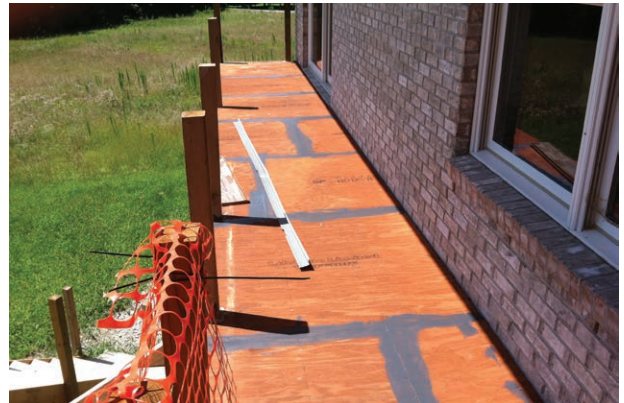
Figure 4. To prevent the plywood joints from telegraphing through the finish, the author filled the joints and other cracks with Bondo and sanded them smooth.
