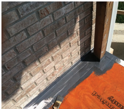
Figure 7. The taped seams and flashed guard posts needed to be embedded with the Super Elasto-Barrier rubberized coating, which the author applied with a brush.
