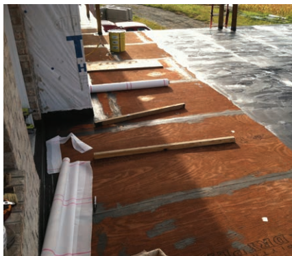
Figure 8. The author then applied the waterproofing to the main roof deck, working in roughly 3-foot-wide sections to correspond to the width of the polyester reinforcing fabric, which comes in 1-meter-wide rolls.
