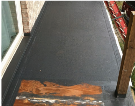
Figure 9. The fabric was laid out over a wet coating, then embedded into additional coating with either a roller or a trowel. It took several coats to build up to the 30-mil thickness recommended by the manufacturer.
