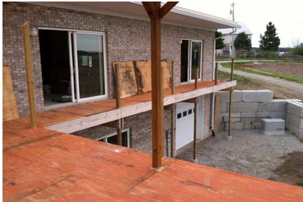
Figure 3. The author applied adhesive to the joists before fastening the \frac{3}{4} -inch T&G plywood to the deck framing with screws.
