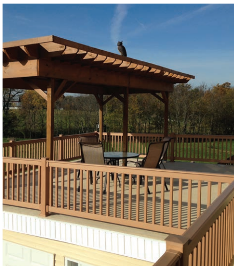
Figure 12. After more than a year in service, the textured deck surface has proven to be durable, stain-resistant, and leak-proof.
