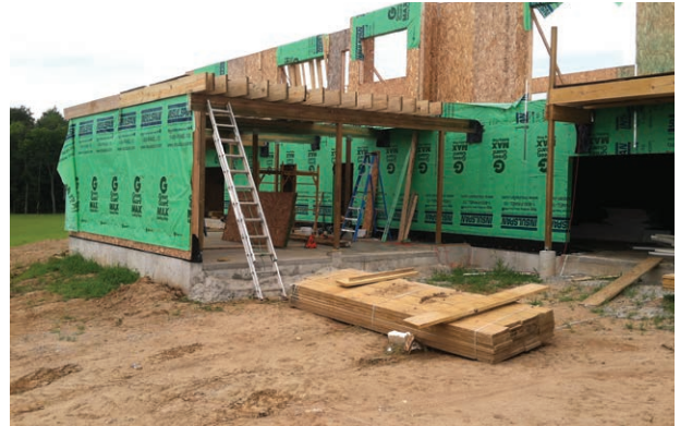
Figure 2. The beams are pitched \frac{1}{4} inch per foot for drainage, and support the roof deck's 2x10 framing.
