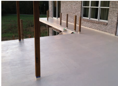
Figure 11. The top coating, available with or without non-skid granules, went on quickly with a roller.
