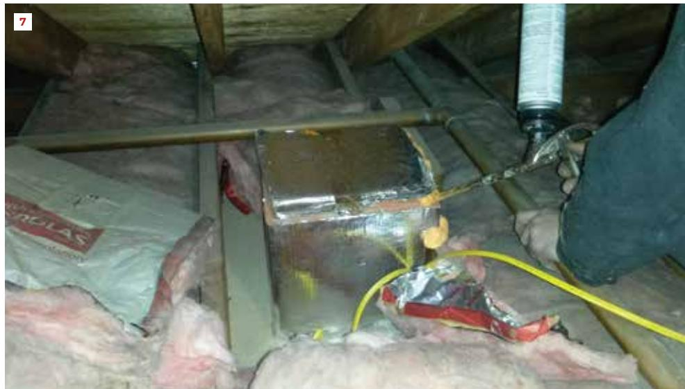
Recessed light fixtures in ceilings (5) are a common source of heat loss in modern homes. When a house is depressurized with a blower door, the infrared scan reveals tell-tale “fingering” as cold air gets pulled along the ceiling (6). Many older can lights of this type are not rated for contact with insulation. In that case, the repair involves building a sealed box of rigid foil-faced insulation around the fixture, making sure the box is large enough to provide the required air space (7).
