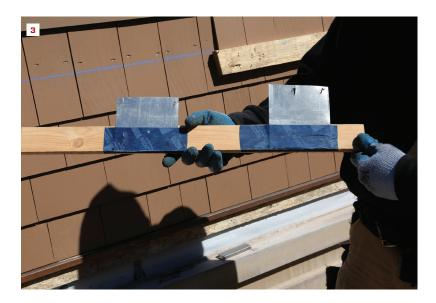
Metal flashing can leave marks as it rubs against the shingles during installation. Short pieces of flashing tape cover the flashing to prevent those marks (3). Keep an eye on the taped flashing and replace the tape as soon as it starts to wear out.
