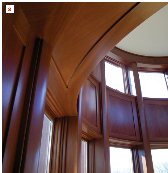
The paint-grade paneling on the first floor (1) and the mahogany paneling on the second floor (2) of this two-story tower (3) on Long Island, N.Y., were made with laminated stiles and rails and 1/4-inch plywood, using the same basic techniques. The plywood fits into a rabbet formed between the laminations in the stiles and rails.
