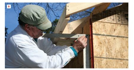
After the subfascia is installed, a line is squared over to locate the ledger for the soffit (5). The ledger is left long to be trimmed when the returns are built (6). Notches under the rafters allow for the use of full-dimension stock on the ends to better support the returns. Blocks made from 2x4s attach to the rafters and to the ledger to support the soffit material and soffit vent (7).
