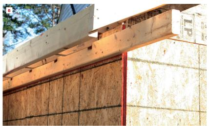
I like to cut the tails from above because the saw kerf opens as the cut nears completion, letting the waste fall harmlessly down and away from the saw.
