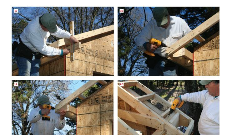
To frame the return, plumb down and cut the ledger to length (17). Then screw a 2-by block to the back of the barge rafter and to the ledger (18). Cut and fill in the triangular piece, keeping the face in plane with the barge rafter and the bottom edge in line with the blocking for the soffit (19). Before the roof sheathing goes on, take advantage of the access to easily attach the return framing and nailers for the rake (20).
