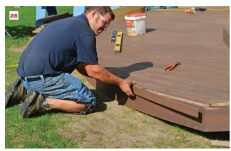
**Roberts trimmed the curved deck edge** using synthetic Fiberon ProTect fascia (23). At 3/4 inch, the composite material is flexible enough to follow the curve. After applying Fiberon decking, he rough-cut the deck boards to the curve with a circular saw, then made a second, finer cut with a jigsaw (24). He smoothed the edge with a router equipped with a flush-cut bearing bit (25), then covered the exposed end cuts with a second trim piece (26).
