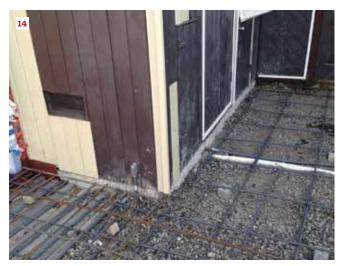
At any of the joints in the pan decking—where concrete might leak through—we used duct tape as a sealer.
