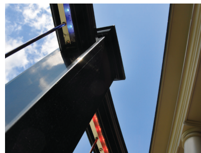
Each low-voltage LED on the flexible strip is capable of displaying red, green, or blue light.
