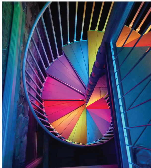
LED strips tucked underneath the nosing of each tread illuminate the staircase.
