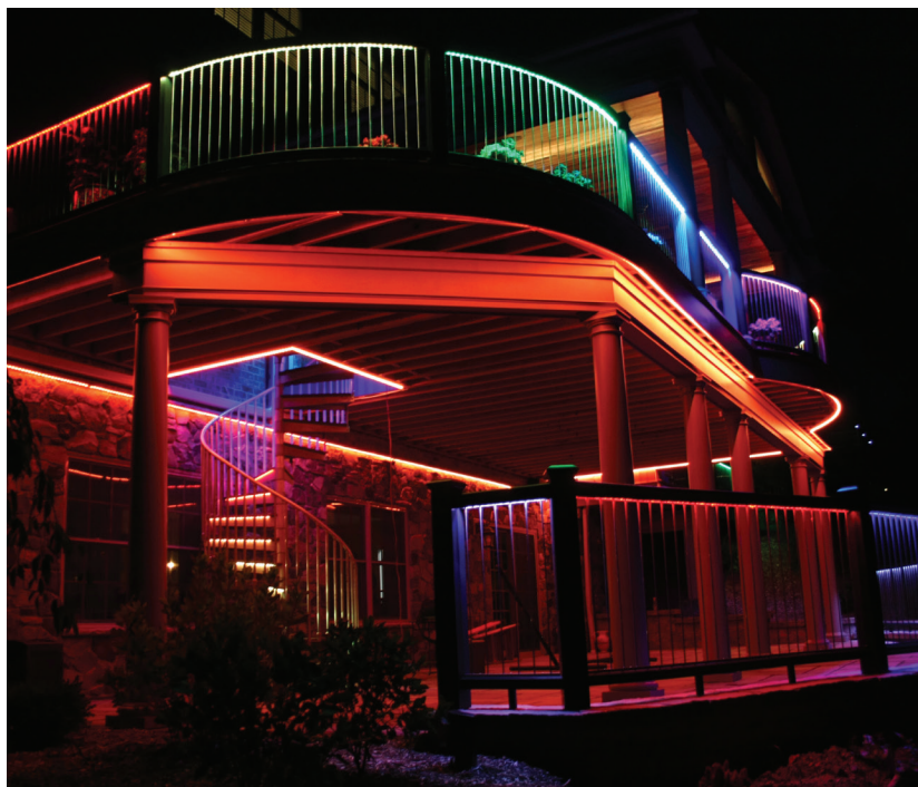
The deck is illuminated by digital RGB LED lighting strips, which have about 10 individually controllable LEDs per foot.
