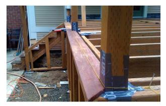
allows the picture-frame-to-field-decking transition to happen in a gap, where there won't be blocking to hold the moisture (see photo, above). I use small 4x4 offcuts to maintain the spacing between posts. This method requires fascia outside of the framing to keep help support the picture rail, but that's easy enough to do; in fact, I usually install spacers between the fascia and the framing to avoid trapping water there and to give the picture rail a stronger connection.
