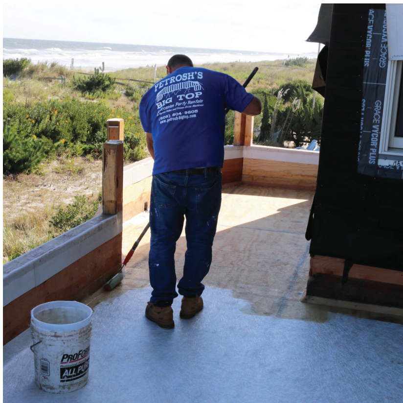
Figure 3. A combination of different applicators, including paint rollers (top) and disposable brushes (bottom) were used to thoroughly saturate the fiberglass mat with resin.
