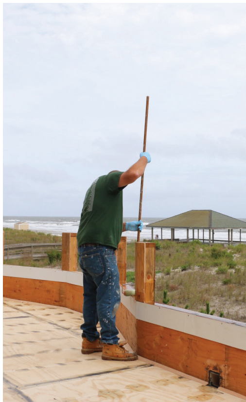
Figure 2. Working from the top down, all the surfaces that would receive the fiberglass covering were primed with a “hot coat” of resin, including the top of the parapet wall (left). After the resin was allowed to cure for a day and then sanded smooth and thoroughly vacuumed, a layer of 1.5-ounce chopped fiberglass mat was spread out over the deck surface (right). Note how the mat extends up the parapet walls, to create a pan.
