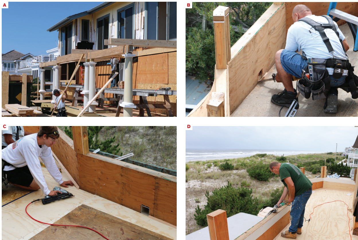
Figure 1. The joists were cut with a taper so that the roof deck would drain toward the perimeter (A). Water drains through scuppers cut into the bases of the parapet walls (B). To ease the transition between the flat roof deck and vertical walls, cant strips ripped with a 45-degree angle were installed in all of the corners (C). In addition to covering the subfloor with smooth 1/2-inch AC plywood underlayment, the crew eased the edges of the parapet wall with a grinder to prep the deck for the fiberglass contractor.
