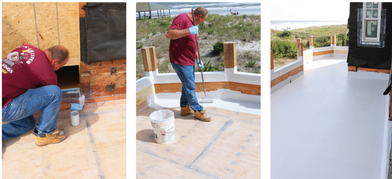
Figure 4. After the lay-up was completed and the resin had cured another day, the fiberglassed surfaces were sanded and then dusted off to prep them for the gelcoat finish. Nooks and crannies were painted with a brush (left), while a paint roller was used to cover larger areas (center). The cured gelcoat (right) provides a durable, weatherproof walking surface, though PT sleepers could also be glued to the fiberglass and standard decking applied for clients who don't like the look or feel of fiberglass.
