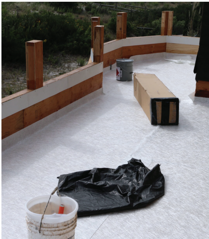
Figure 2. Working from the top down, all the surfaces that would receive the fiberglass covering were primed with a “hot coat” of resin, including the top of the parapet wall (left). After the resin was allowed to cure for a day and then sanded smooth and thoroughly vacuumed, a layer of 1.5-ounce chopped fiberglass mat was spread out over the deck surface (right). Note how the mat extends up the parapet walls, to create a pan.
