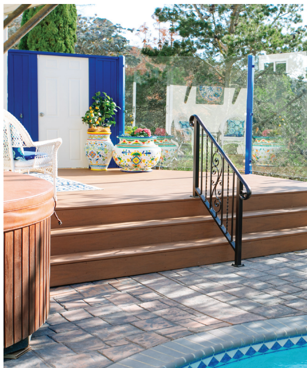
Figure 3. Although the new concrete slab is important structurally, it has a decorative colored and stamped finish, flush with the original coping around the gunite pool (top). Partially cantilevered steel framing supports the new composite deck at one end of the pool (above).
