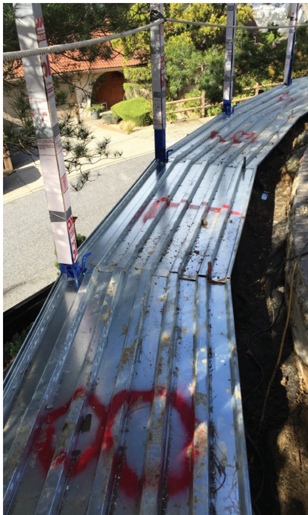
Figure 2. After the guard posts were welded to the columns, workers cut and fit the B Formlok galvanized steel panels that would support the cantilevered portion of the new concrete slab (top left). A pour stop of 1/4-inch-by-6-inch steel welded to the posts forms the edge of the slab (bottom left).
