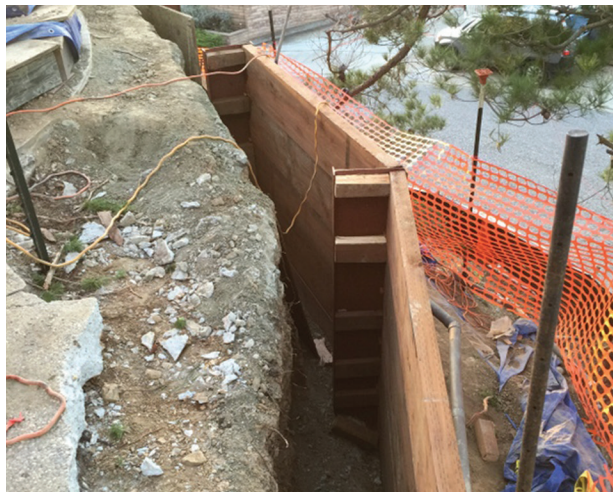
Figure 1. The existing concrete slab flanking the edge of the pool was demolished to expose the steel columns supporting the retaining wall. Blocks held the new 3x12 PT timber laggings in place until the excavation could be backfilled (top left). The prefabricated guard-post assemblies were temporarily clamped in place, then welded to the columns (center left). Horizontal steel tubes welded to both the columns and the guard posts stabilized the posts and helped support the Formlok panels when the concrete was poured (bottom left).
