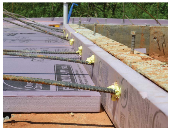
Two inches of insulation at the slab edge and under the slab shaved 8,000 Btu/hour off the heating load of this Atlanta slab on grade.
