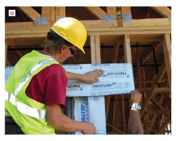
With the side flashings in place (7), the window unit can be installed. (To meet the window manufacturer's requirements, the window flange must be installed in a bed of sealant; see "Installing Flanged Windows," Jan/16.)
