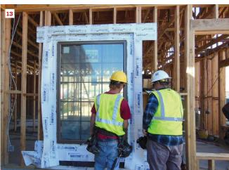
The final membrane flashing is slit at the edges of the opening and folded inwards across the horizontal head and down over the window flange (12), completing the flashing assembly (13).
