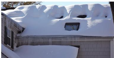
Code requires roofs to be strong enough to carry the weight of live loads such as the weight of workers and stacked up materials (top), and snow loads (above) in areas that receive significant snowfall.
