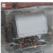
Left: This site-made metal flashing (13) is less reliable than a factory-built one. Factory boots for these vent pipes (14) are reliable and easy to install. A factory EPDM collar for this plumbing vent (15) is more reliable than a site-made flashing. Rectangular penetrations (16) are flashed using skylight details, with overlapping layers of flexible flashing tape.
