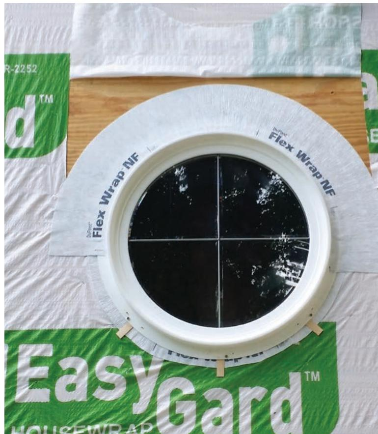
A flexible butyl-based flashing material works well for flashing round-top windows, but the sill is tricky. In this case, the installer has left the bottom uncaulked and added shims to promote drainage.
