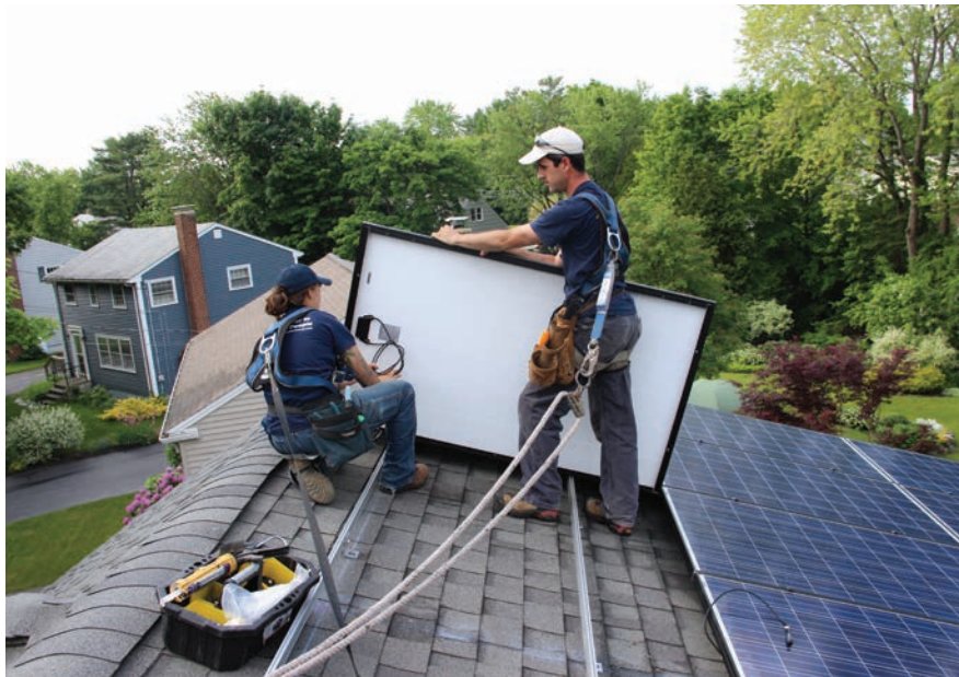
Technicians for Revision Energy install PV panels for a grid-tied system on a Portland, Maine, roof in 2014. A panel array this size might supply all the power a house needs on a net annual basis, but still requires a grid connection to balance surplus summer production against nighttime and winter power needs.
