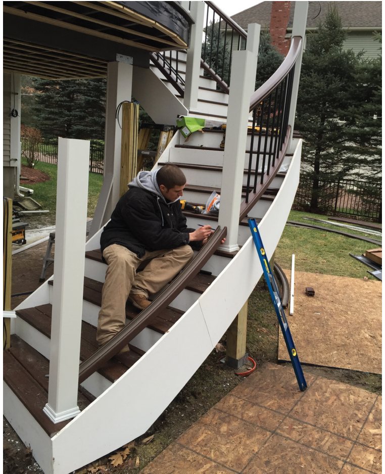
Figure 9. Rail sections also had to be heat-formed to match the radius of the curved stairs. The 16-inch-wide stair skirts were ripped from \frac{3}{4} -inch-thick PVC sheet goods.
