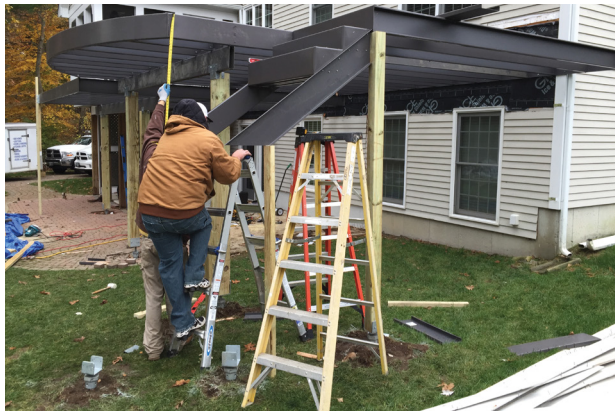
Figure 3. A Trex Elevations stair-stringer assembly consists of both a track (shown being installed) and a matching stringer joist, which will be fastened over the track.
