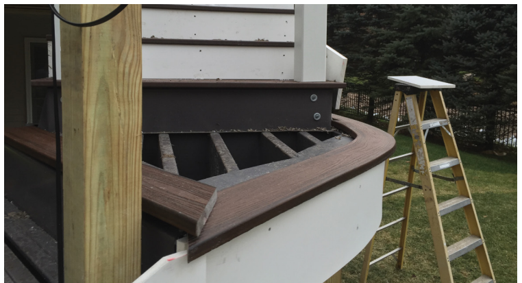
Figure 7. The author used a heating box and a bending table to heat-form the decking for the landing to the proper radius.
