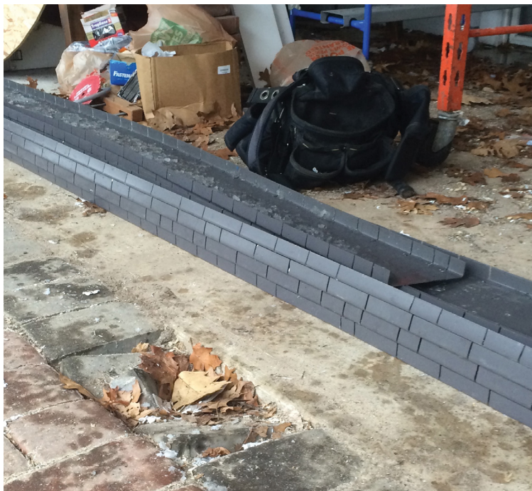
Figure 1. In order to bend the steel framing, the author cuts evenly-spaced kerfs in the upper and lower webs using a circular saw equipped with a ferrous steel blade.
