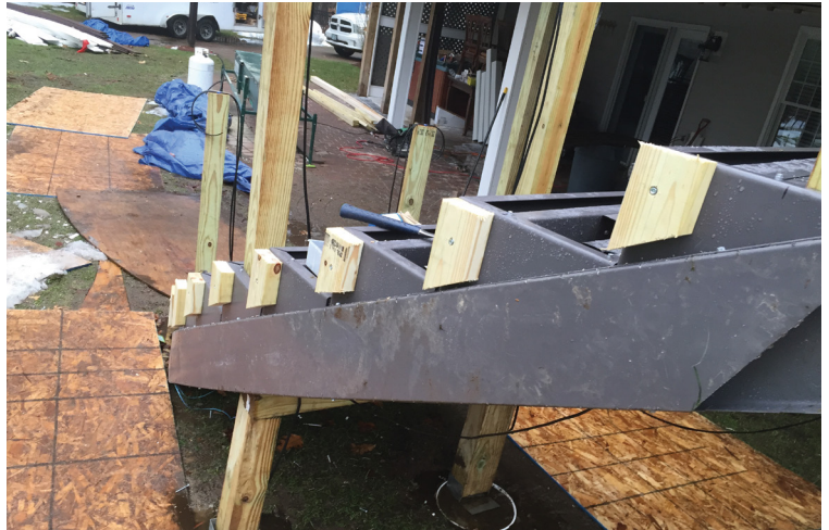
Figure 6. Here, an Elevations joist has been fastened over the stringer track to strengthen the assembly, and blocking has been installed for the PVC trim that will be used to finish the stair.
