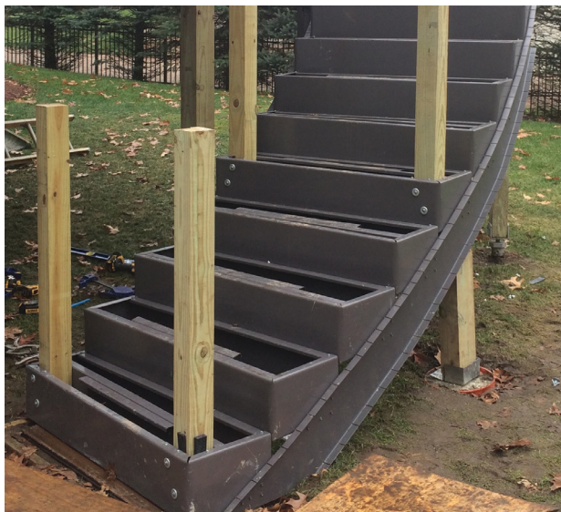
Figure 5. The lower run of stairs curves to match the curve of the deck. The stringer tracks needed to be kerfed so that they could be bent to the proper radius.
