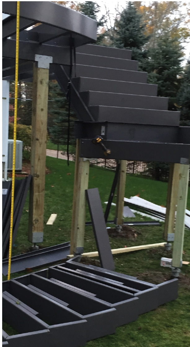
Figure 4. The author prefabricated the stair boxes in his shop using folded sections of track. The boxes are then screwed to the stringers.
