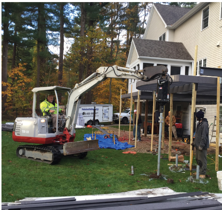
Figure 2. Like the steel-framed deck itself, the landing for the curved stairs is supported by helical piles.
