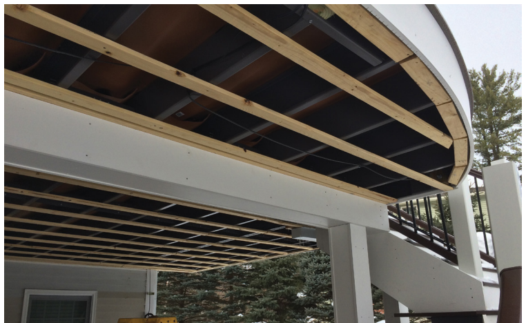
Figure 8. Kerfs cut into the back of the PVC fascia allow it to be bent without breaking, especially in colder weather.
