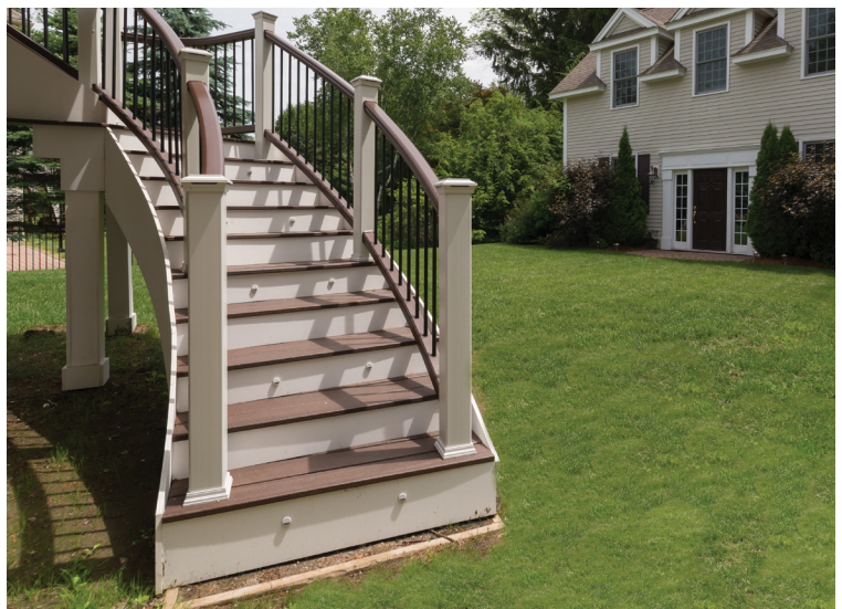
Figure 10. After filling the fastener holes with Cortex plugs, workers gave the trim a final hand-sanding with #220-grit sandpaper.
