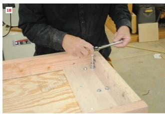
The table-saw stand and worktable starts with a 2-by frame pocket-screwed together (15). Backer blocks at each end will support the clamp track (16). Center the frame on the top and attach it with pocket screws (17). The overhang helps with clamping work to the table. Lay out the track the same as with the miter-saw stand, and attach it with nuts and bolts (18).
