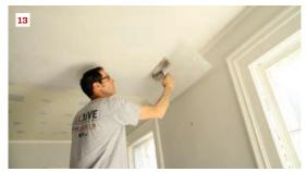
ceiling joists with strips of ½-inch drywall (8) before installing large pieces of the same material to fill in the hole. Note that the plaster around the perimeter should be well secured with screws and plaster washers, and any small areas of exposed lath should also be secured.
