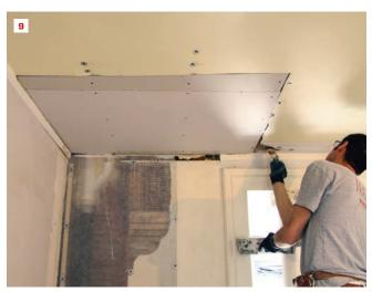
later in this article. For the wall repair, I stapled the fabric over the opening in the wall (3), and then covered it with wire lath, securing the lath with screws and plaster washers (4). As luck would have it, the opening I was repairing could be covered with a single sheet of lath measuring 8 feet by 27 inches—a common size for wire lath.
