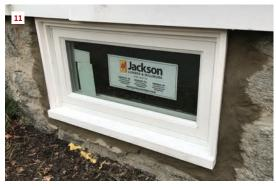
elastomeric latex sealant) onto the front side of the stops and pressed the window against the stops, leaving equal space along both sides for insulation (7).
