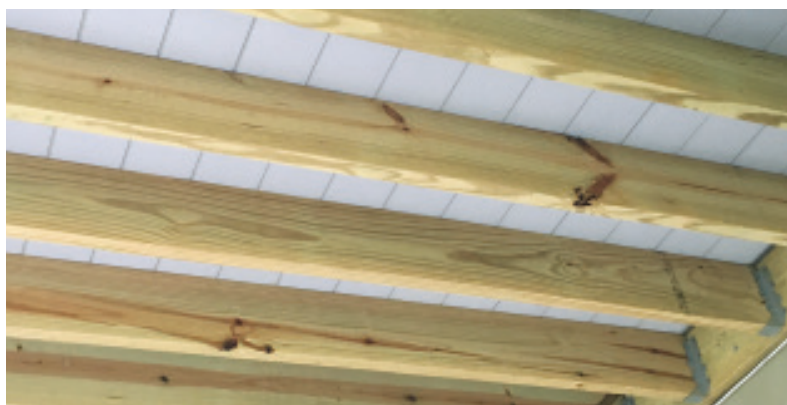
Figure 3. Admiral SpaceMaker is a capped solid-core plank with a built-in silicone edge gasket (center). Before the fasteners are driven into the joists, a BoWrench ( cepcotool.com ) or even a flat-head screwdriver can be used to pry the decking in place, which compresses the gasket (top). The installed decking also creates a bright ceiling for the space underneath (bottom).
