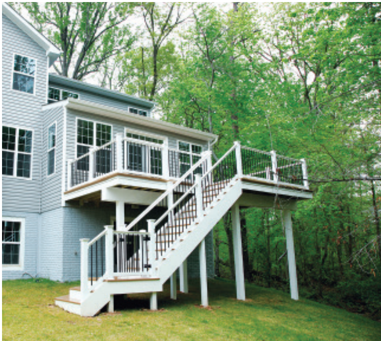
Figure 5. A SpaceMaker deck is ready for phase two: a patio and hot tub on the lower level. Deck framing needs to be sloped with at least a \frac{1}{8} -inch-per-foot pitch for drainage, a consideration when you're retrofitting an existing deck with a waterproof decking product.
