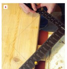
Continue moving the square up the side of the stringer and tracing the steps until you have marked the proper number of rises—in this case, four (3).
