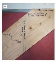
Draw in all of the details for the bottom of the stair, including the tread and riser materials and flooring, both existing and planned (5). If you don't know whether the stairs are going in before or after the finished floor, label both options clearly.
