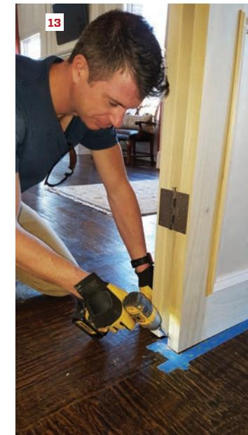
After scribing the stationary panels to fit, the author routs the hinges for the operable panels (10). The stationary panels screw to the jamb and to the top free corner (11). He scribes and mounts the operable panels and aligns their free edges by pushing lightly at the bottom of the stationary panel (12). When they line up, the bottom free edges are anchored in their adjusted positions (13).
