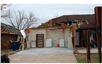
This garage door opening (12) shows a classic racking failure that is also commonly seen in earthquakes. Image (13) shows similar racking of another garage door frame, plus catastrophic failure of the adjacent walls and roof—likely a result of the sudden pressurization of the building when the garage door was lost. In images (14) and (15), pressurization of the garage apparently contributed sufficient force to cause the loss of roof sheathing in nearby areas of the main house roof.
