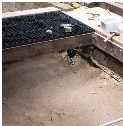
Figure 3. Standard deck framing was used to support Silca Systems grating and stone pavers. Note the SST HD2A holddown connectors and the robust cross-bracing, a precaution against seismic activity (far left). Silca Systems plastic grates are light and easy to cut, and they attach to the deck framing with four screws, one in each corner (left).
