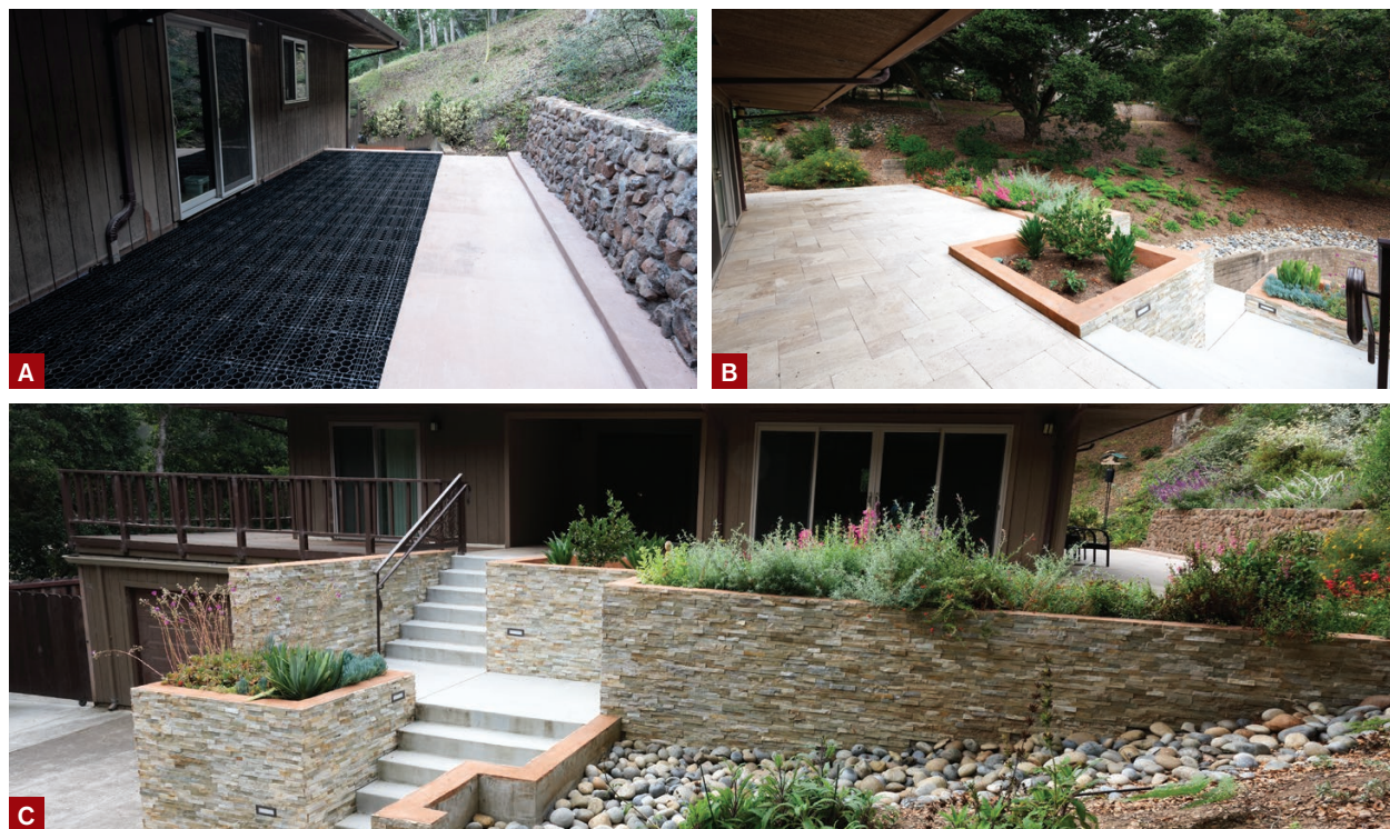
Figure 4. Prior to installing the 1 \frac{1}{4} -inch-thick travertine stone pavers, the author applied an isolation membrane to the slab. The pavers over the slab were set in thinset mortar, and the rest were simply glued to the grating with construction adhesive (A). The pavers were set in a Versailles pattern, which is commonly used for indoor tile installations (B). The new deck features wider stairs and landings for easier access, more outdoor living area, and improved drainage on the sloped site (C).
