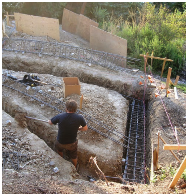
Above, a worker shovels out the trench for grade beams that will support the stem wall for the unconditioned crawlspace under Sylvia Wallis' addition.
