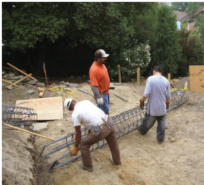
Above, foundation workers set rebar cages for deep structural piers into the hillside for Sylvia Wallis' high-performance addition.
