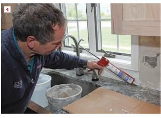
**Prepping the backsplash.** The author begins by screwing a temporary ledger to the wall behind the stove to support the tile (1). For the mural that will be installed above the stove, he does a dry layout first, cutting the mosaic sheets to fit inside a mitered border (2). Drywall patches bedded in thinset fill the holes left over from relocated outlets (3). Behind the sink, a bead of silicone seals the seam between the tile and the countertop (4).
