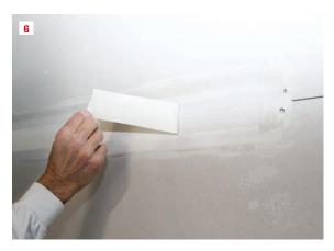
Embedding the tape. With the tape positioned over the seam, the author draws his taping knife along the length, holding the knife at a steep 60-degree angle while pinning the tape in place with the trowel he uses to carry compound (4). He tests the embedded tape (5); if it leaves a dimple, not enough mud has been forced from the back of the tape. You can also peel back the end of the tape to inspect (6): There should be an even layer no more ½ inch thick.
