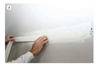
First coat. For hand-taping, there are three options for carrying mud (1)—a hawk (left), a large trowel (center) or a pan (right). The author uses a 6-inch knife for the first coat (2), applying a healthy ½-inchthick bed of compound on the seam. He coats the entire length (up to about 20 feet) before rolling out the tape and gently pressing it into the mud every 18 inches or so to keep it in place (3).
