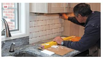
Tiling the second backsplash wall. Tile layout for this wall begins with a full tile at the window casing, where the tile will be the most visible (8). Odd sizes won't be nearly as noticeable in the corner under the cabinets. The installation continues from that first tile toward the corner (9). Then, after the author installs the mosaics under the window casing and behind the sink, he works from the other side of the window over to the opposite corner (10).
