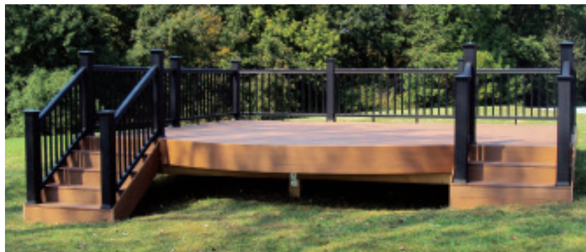
Guardrails aren't required but may be a good idea on decks less than 30 inches above the ground. Stairs with four or more risers require at least one handrail.
