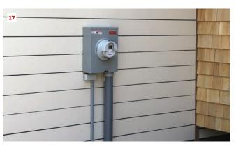
Exterior outlets mount into boxes that are flashed into the drainage plane (14) and the rainscreen mesh. Shingles then complete the outer weather barrier (15). Temporary strapping the thickness of the siding holds the electric meter out from the strapping and the drainage plane (16) until the siding is installed. The meter then attaches directly to the siding, keeping the drainage plane intact behind the meter (17).
