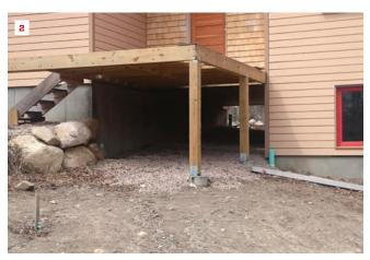
A ground gutter (above) channels water from the perimeter of a house before it can collect and compromise the foundation. A depression or swale sits below the drip line of the roof. Water seeps through filter fabric and crushed stone before entering a pipe that carries it away safely.
