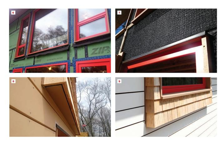
Strips of building paper that will be integrated with the building-paper drainage plane provide additional protection for the window sills (6). Certain wall areas are shingled in cedar for a visual accent. Rainscreen mesh applied over the building paper provides drainage space behind the shingles (7). The mesh extends to the bottom of the rainscreen to provide a measure of ventilation for the siding, as well (8), and transitions between the two types of siding have to be carefully detailed (9).
