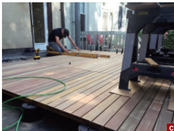
Figure 2. The 2-foot-by-4-foot ipe deck panels are flush with the top of the ipe curb and are supported by Bison Versadjust pedestals located at the corners and midpoints of the panels (A). To account for the slope of the roof, the author used different sizes of pedestals, each with a range of adjustment. The pedestals have angled bases that can be rotated to provide a perfectly flat surface to support the deck panels (B). During installation, spirit levels were used to level the deck panels, while tabs fitted to the tops of the pedestals provided the proper spacing between panels (C).
