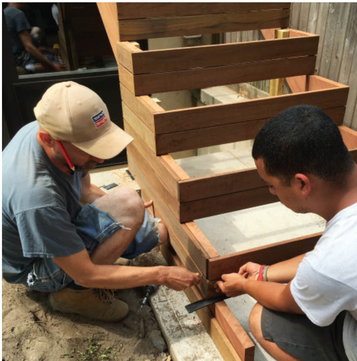
Figure 4. The stair stringers were cut from 2x12 mahogany, while the risers, treads, and trim were crafted from 1x4 ipe.
