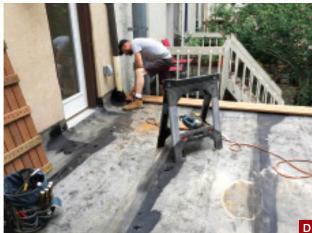
Figure 1. Working on top of the temporary roofing membrane, project manager Danny DoCouto began by installing the first of four layers of 2x10 SPF around the perimeter of the roof to create a curb (A). Because the curb establishes the final elevation for the rooftop deck, great care was taken to shim the second 2x10 layer so that it would be absolutely flat and level in every direction (B). Once the 6-inch-high curb was completed, a roofing contractor installed tapered insulation panels to provide drainage, \frac{3}{4} -inch CDX plywood underlayment, and then two layers of torch-down modified bitumen roofing membrane (C). The curb is capped with \frac{5}{4} x12 ipe that's face-screwed to the curb with countersunk stainless steel fasteners. To help make the assembly watertight, the ipe is bedded in sealant (D).
