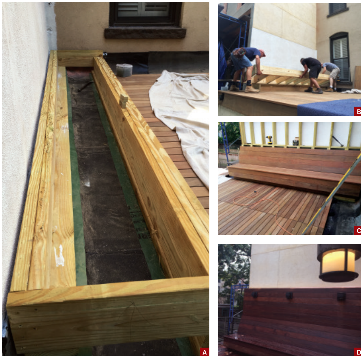
Figure 3. The PT base for the nearly full-width bench rests on sleepers, which are separated from the membrane roofing with strips of thick plastic (A). No fasteners could be used to anchor the bench to the wall behind it, which belonged to the neighboring brownstone residence (B). The bench was finished with 1x6 ipe (C) and fitted with lighting fixtures (D).
