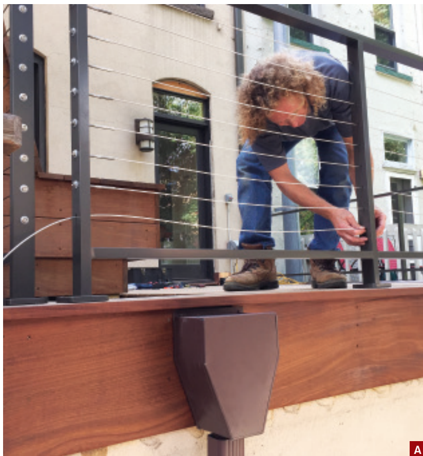
Figure 5. Water runs off the deck through a large scupper in the curb and drains through a custom-fabricated leader head. The powder-coated aluminum deck railing is also custom-fabricated (A). Note the conduit for electrical wiring that runs underneath the deck panels, past a new door that was part of this project, to the bench lighting (B). The new rooftop deck creates a comfortable backyard outdoor living space, a valuable commodity in urban New Jersey (C).
