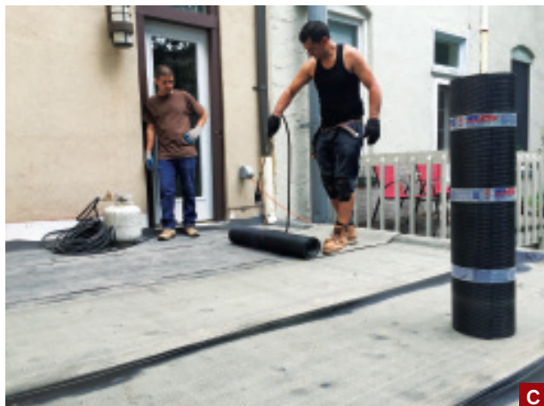
Figure 1. Working on top of the temporary roofing membrane, project manager Danny DoCouto began by installing the first of four layers of 2x10 SPF around the perimeter of the roof to create a curb (A). Because the curb establishes the final elevation for the rooftop deck, great care was taken to shim the second 2x10 layer so that it would be absolutely flat and level in every direction (B). Once the 6-inch-high curb was completed, a roofing contractor installed tapered insulation panels to provide drainage, \frac{3}{4} -inch CDX plywood underlayment, and then two layers of torch-down modified bitumen roofing membrane (C). The curb is capped with \frac{5}{4} x12 ipe that's face-screwed to the curb with countersunk stainless steel fasteners. To help make the assembly watertight, the ipe is bedded in sealant (D).
