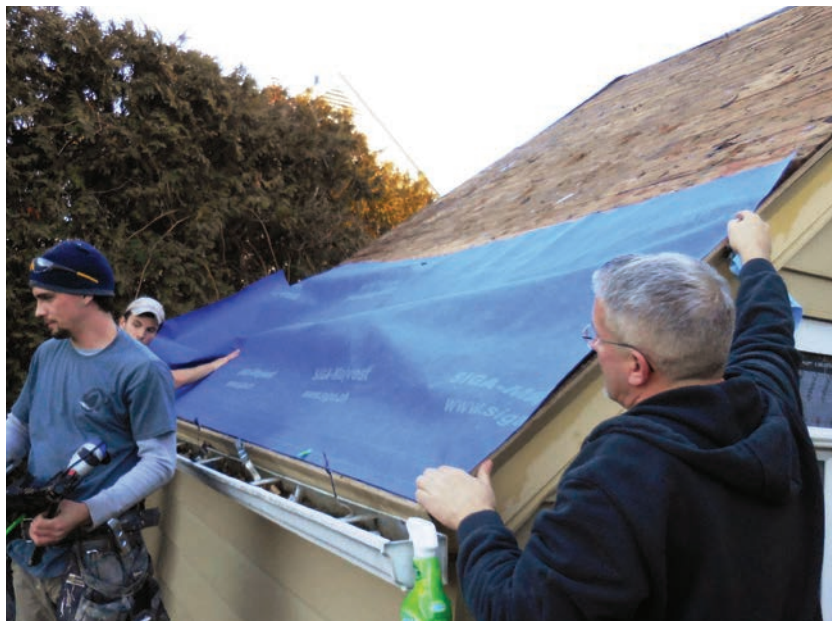
The author and his crew spread Majvest weather barrier membrane over the original board sheathing of the roof. With a perm rating of at least 34, Majvest is vapor open, but it resists driving rain.
