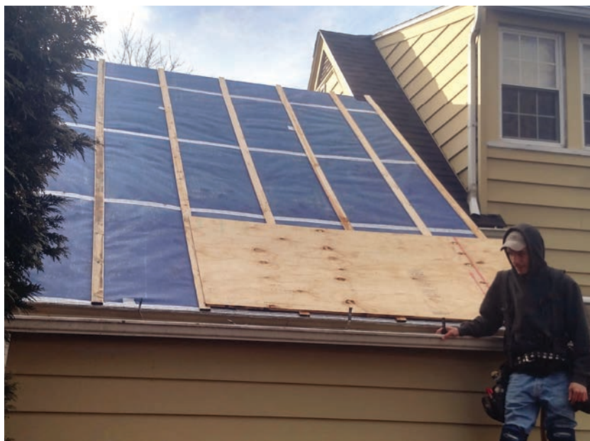
The crew installs plywood roof sheathing over \frac{3}{4} -inch wood strapping as a nailbase for asphalt shingles. This creates an air space that will allow moisture diffusing out of the cathedral roof to escape the assembly through convection.
